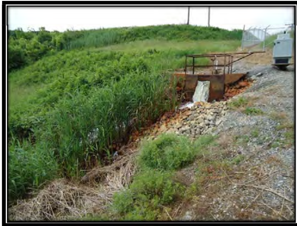
Photo 26 – Outlet Structure from Ash Pond 4 May 25, 2011 IL50160
