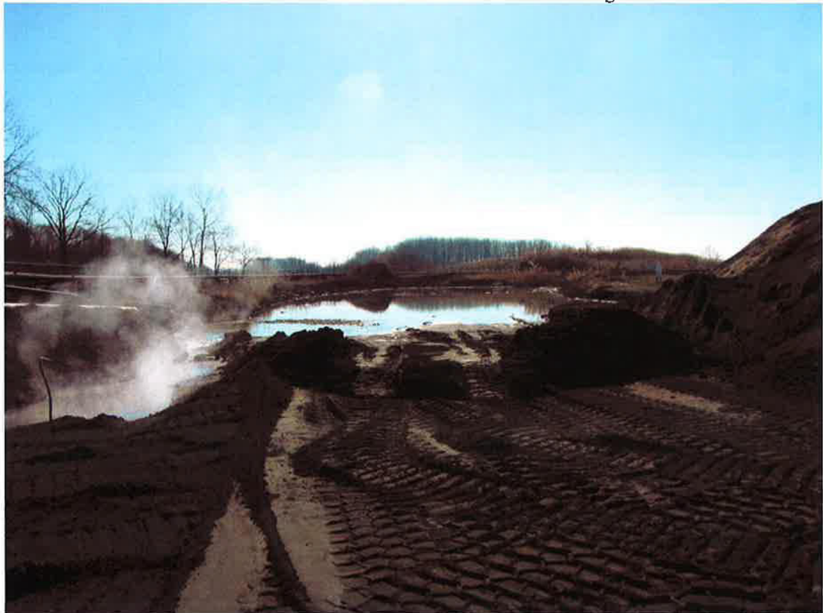
Photo #12 – Bottom Ash Pond – North end looking south
