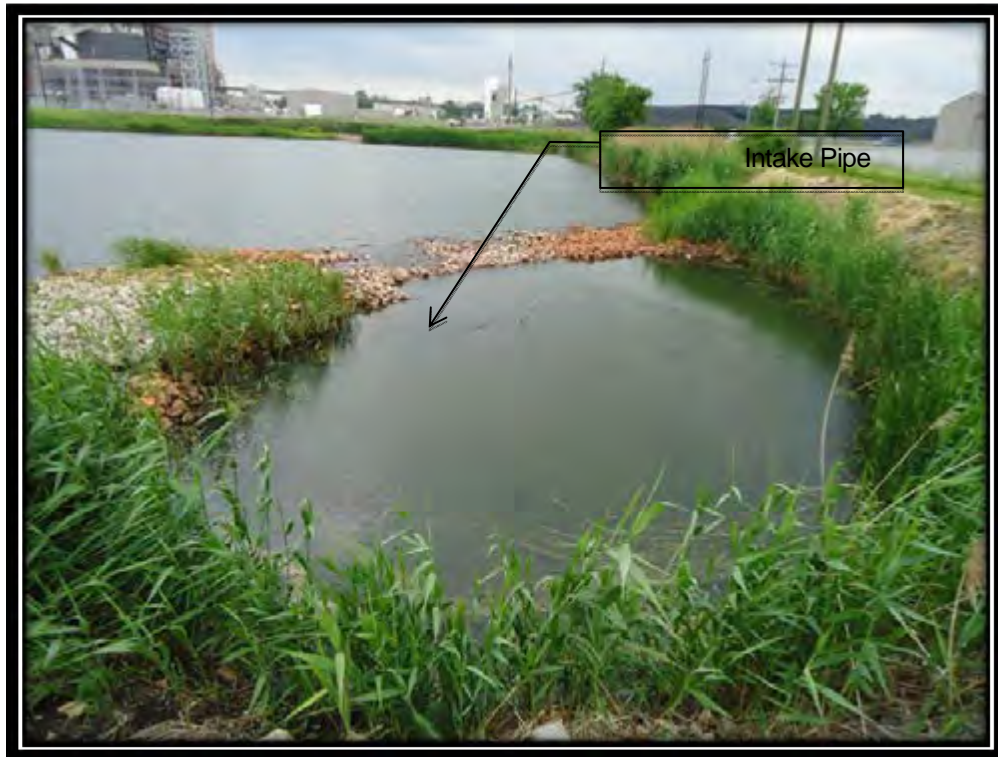
Photo 22 – Intake from Pond 4 to Outlet Structure
