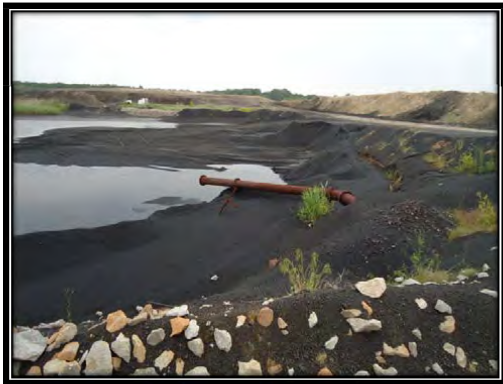
Photo 10 – Ash Pond 2 Inlet Sluice Pipe May 25, 2011 IL50160
