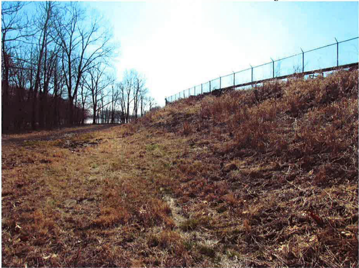
Photo #11 – Bottom Ash Pond – Northeast berm looking south
