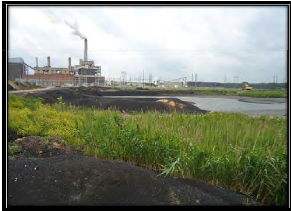
Photo 7 – Ash Pond 2 General Conditions Photograph May 25, 2011 IL50160
