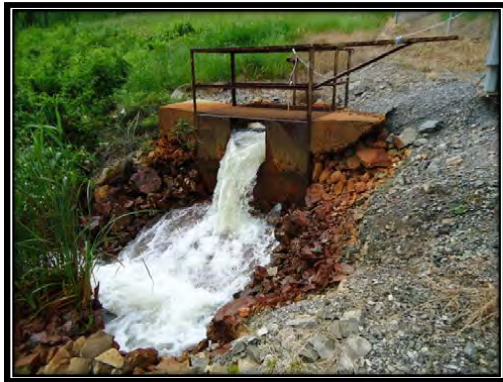
Photo 24 – Outlet Structure from Ash Pond 4
