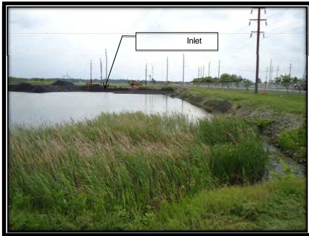
Photo 14 – Ash Pond 1 General Conditions Photograph (Note Inlet Sluice Pipe) May 25, 2011 IL50160
