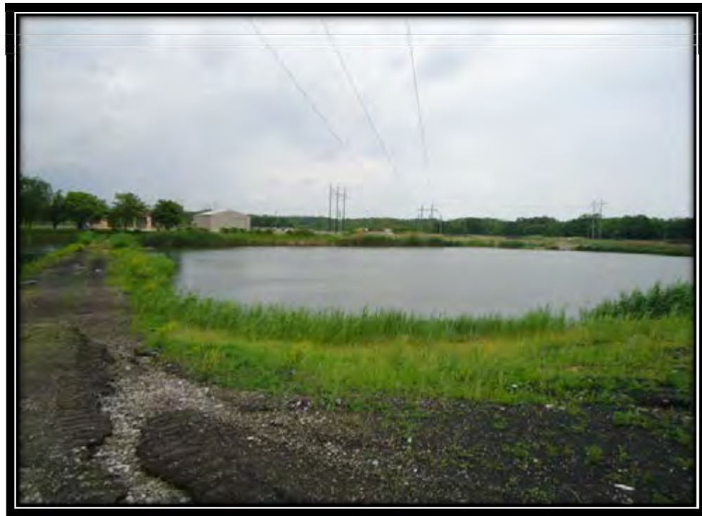
Photo 19 – Pond 4 General Conditions Photograph
