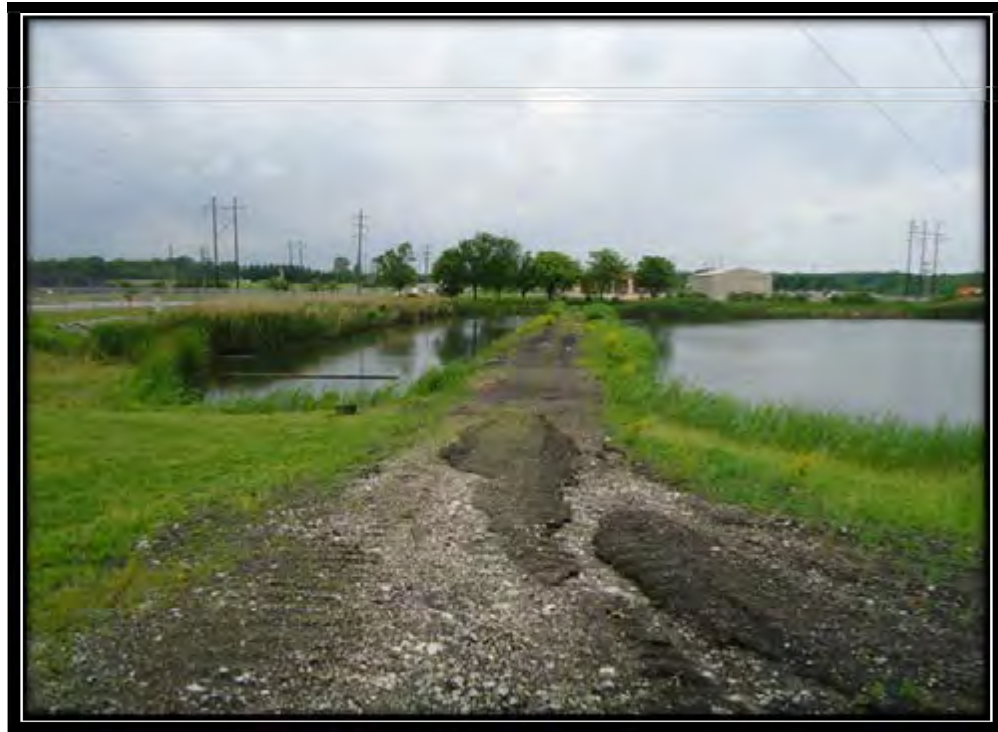
Photo 17 – Pond 4 General Conditions Photograph
