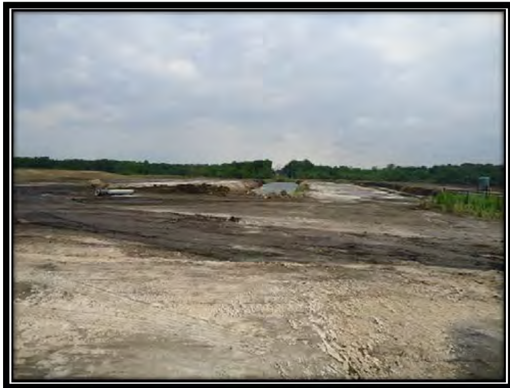
Photo 6 – Pond S-3 General Conditions Photograph
