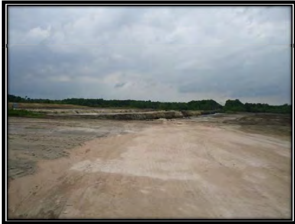
Photo 4 – Pond S-2 General Conditions Photograph
