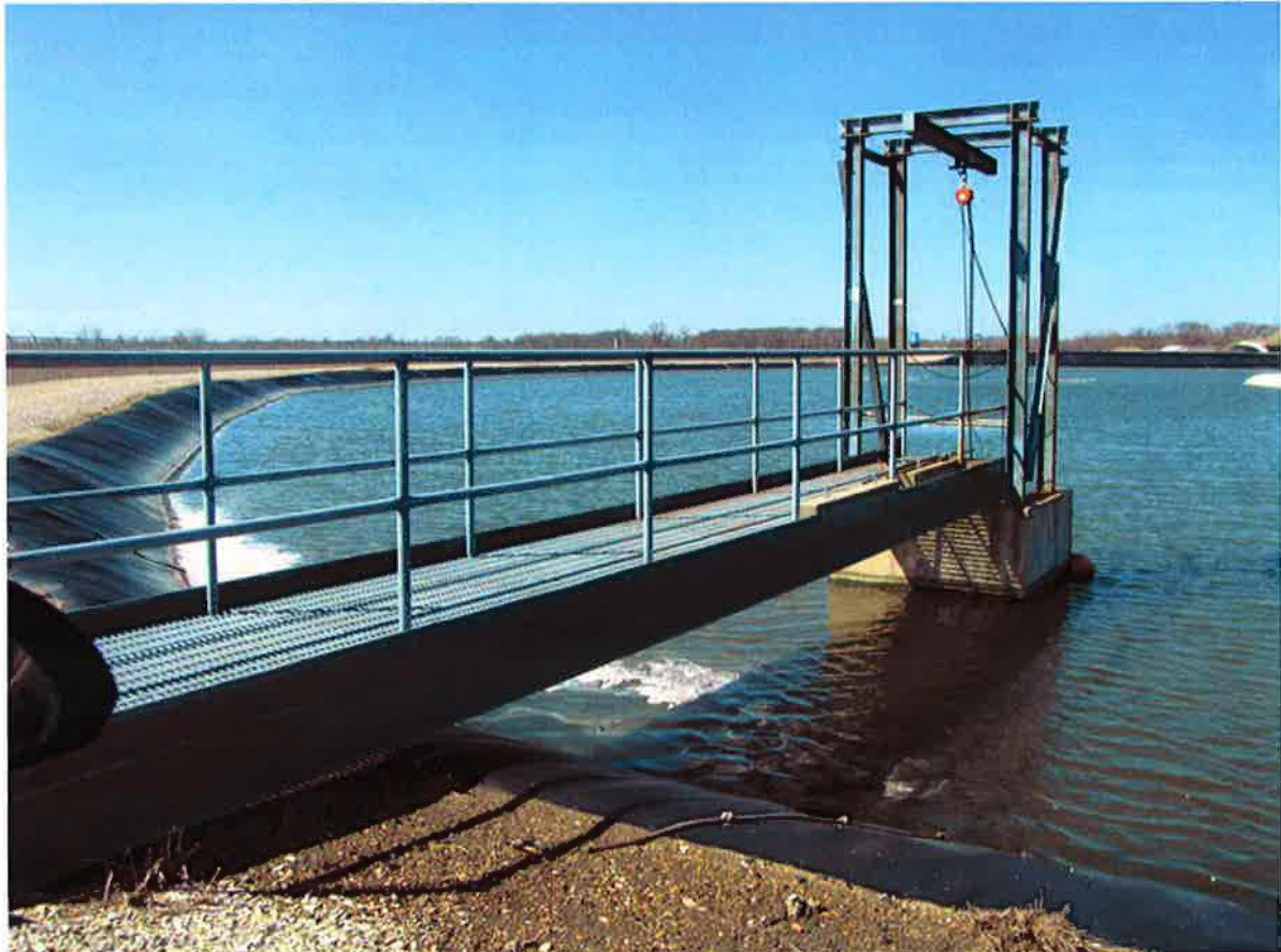
Photo #6 – Ash Pond B – Outlet structure
