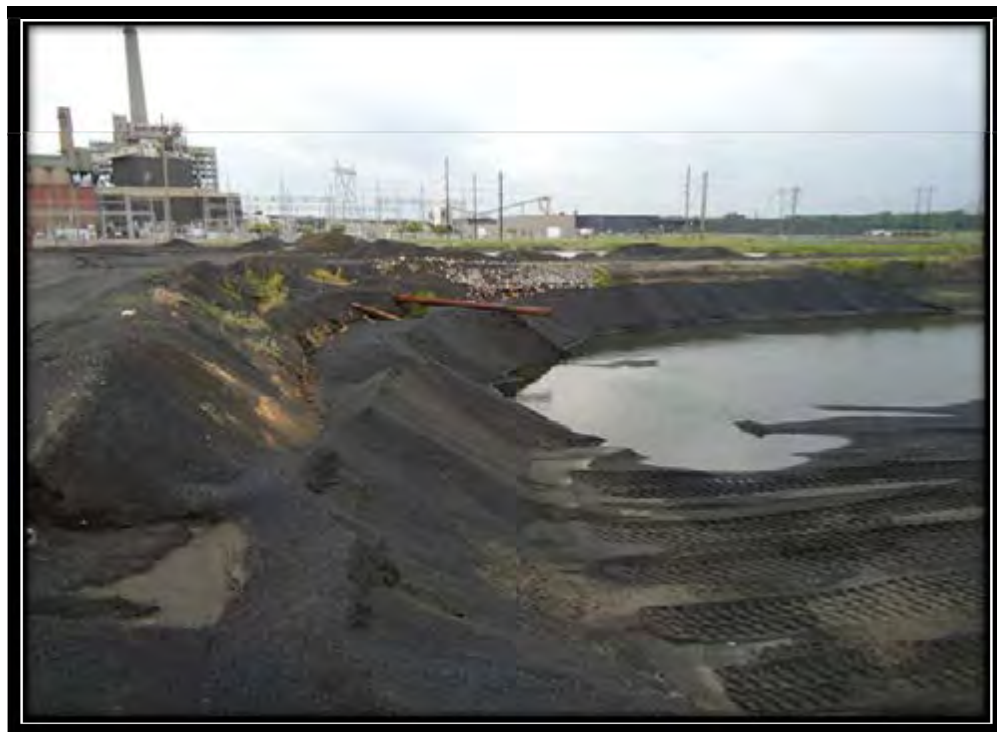
Photo 9 – Ash Pond 2 Inlet Sluice Pipe May 25, 2011 IL50160
