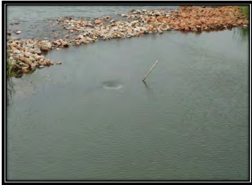
Photo 23 – Intake from Pond 4 to Outlet Structure (note submerged pipe)
