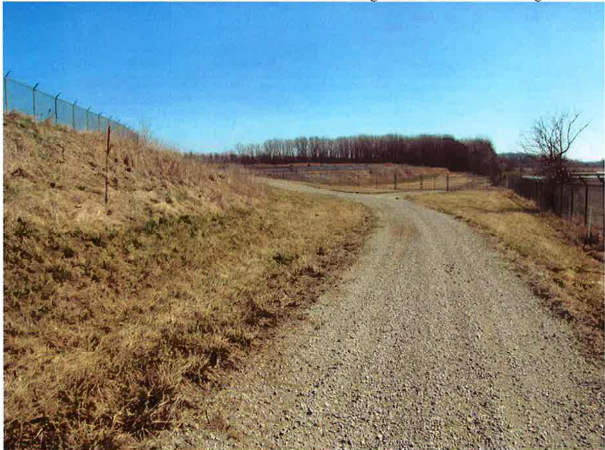
Photo #8 – Ash Pond B – South embankment looking west to Pond D in background
