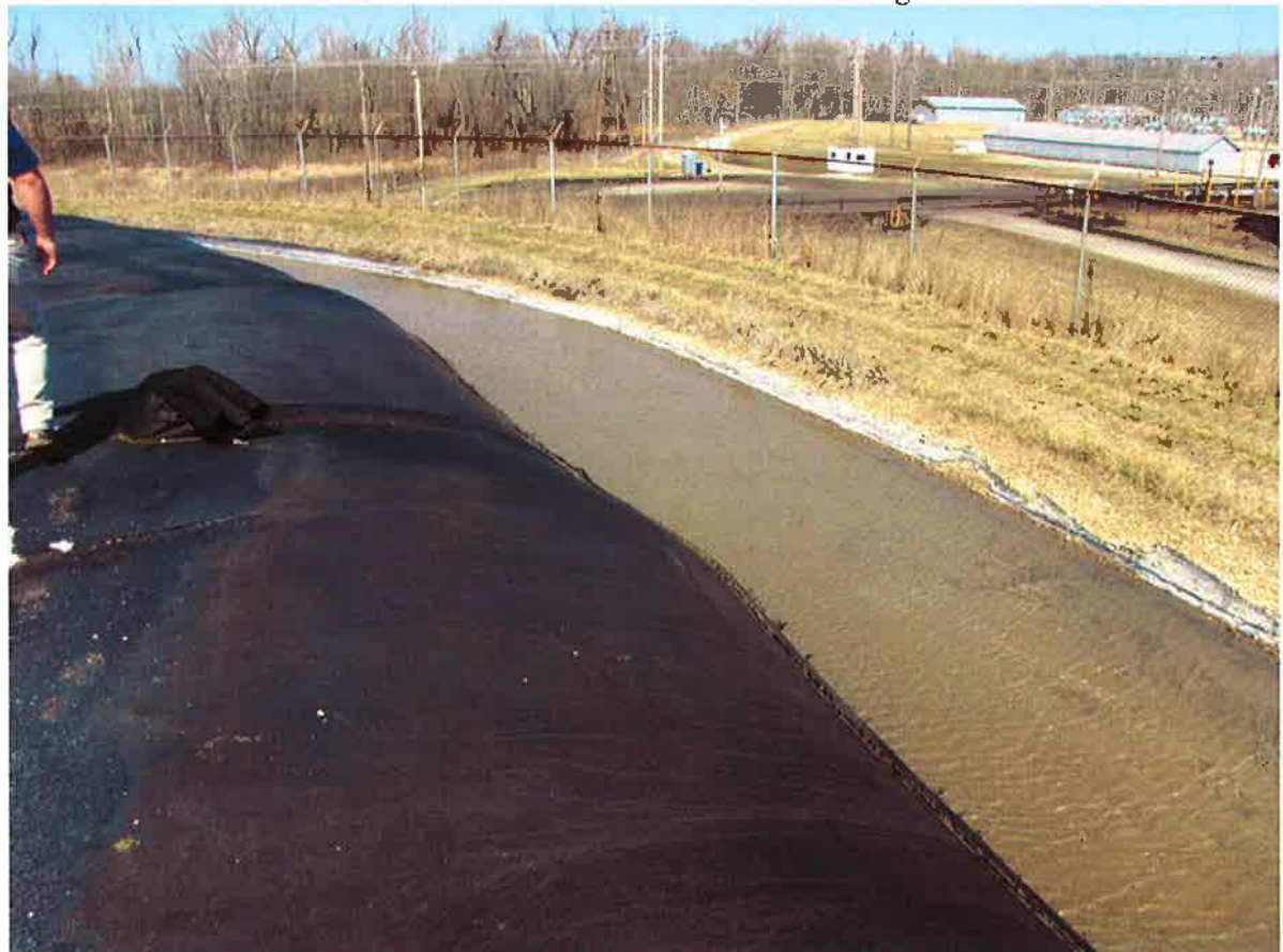
Photo #2 – Ash Pond A – East berm looking north
