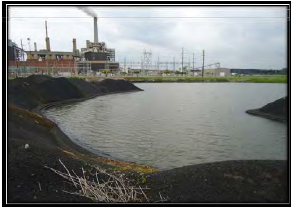
Photo 11 – Ash Pond 1 General Conditions Photograph May 25, 2011 IL50160
