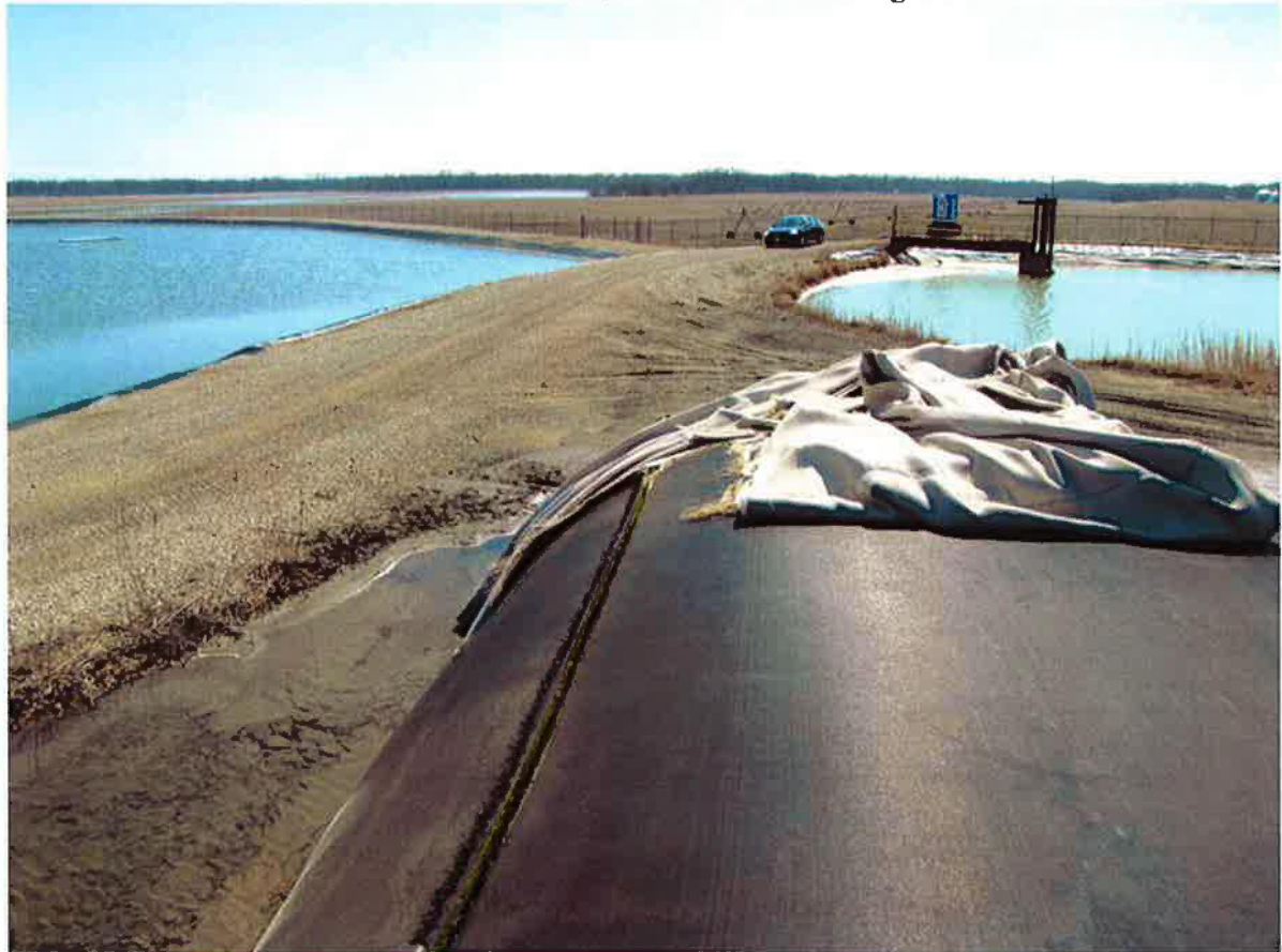
Photo #4 – Ash Pond A - East berm looking south
