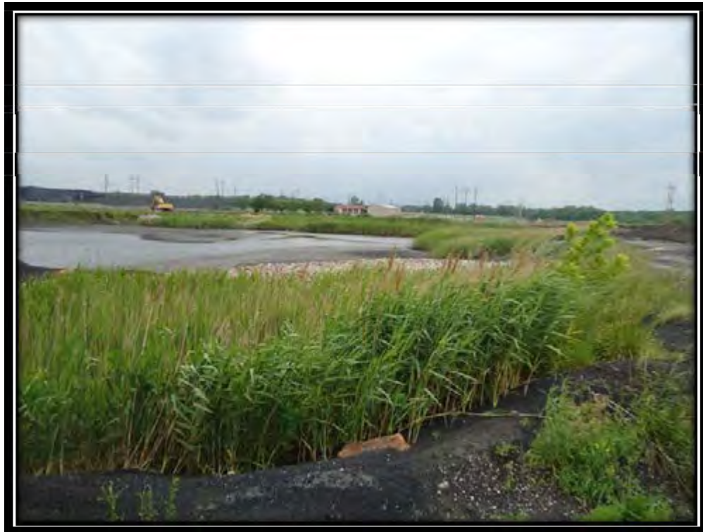
Photo 8 – Ash Pond 2 General Conditions Photograph May 25, 2011 IL50160
