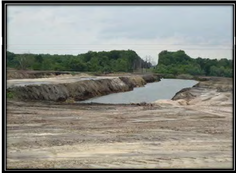
Photo 5 – Pond S-2 General Conditions Photograph
