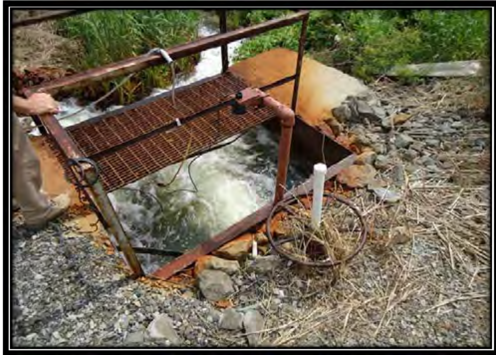
Photo 25 – Outlet Structure from Ash Pond 4 May 25, 2011 IL50160
