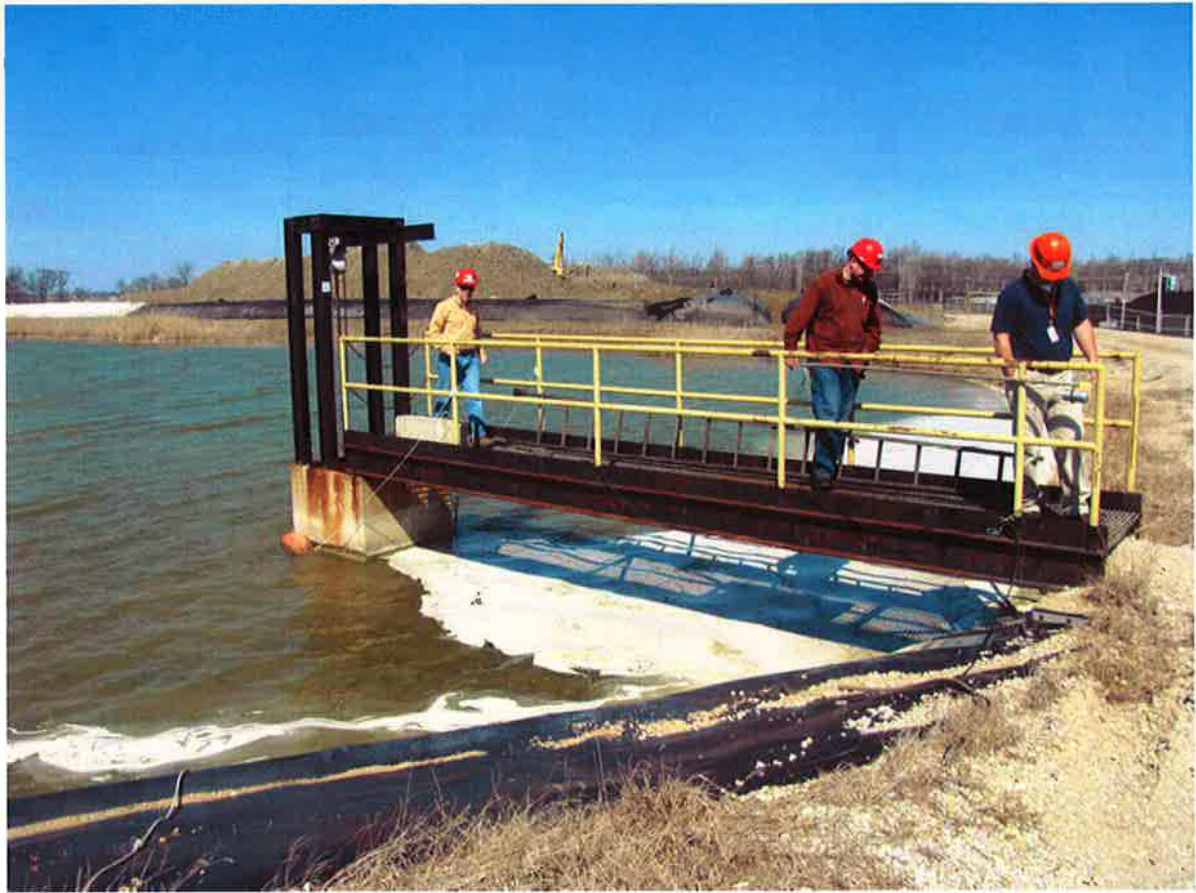
Photo #5 - Ash Pond A – Outlet structure
