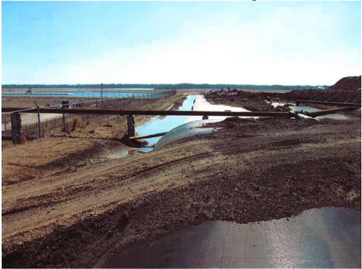
Photo #3 – Ash Pond A – East berm looking south
