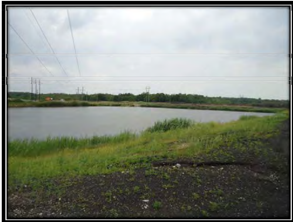
Photo 18 – Pond 4 General Conditions Photograph
