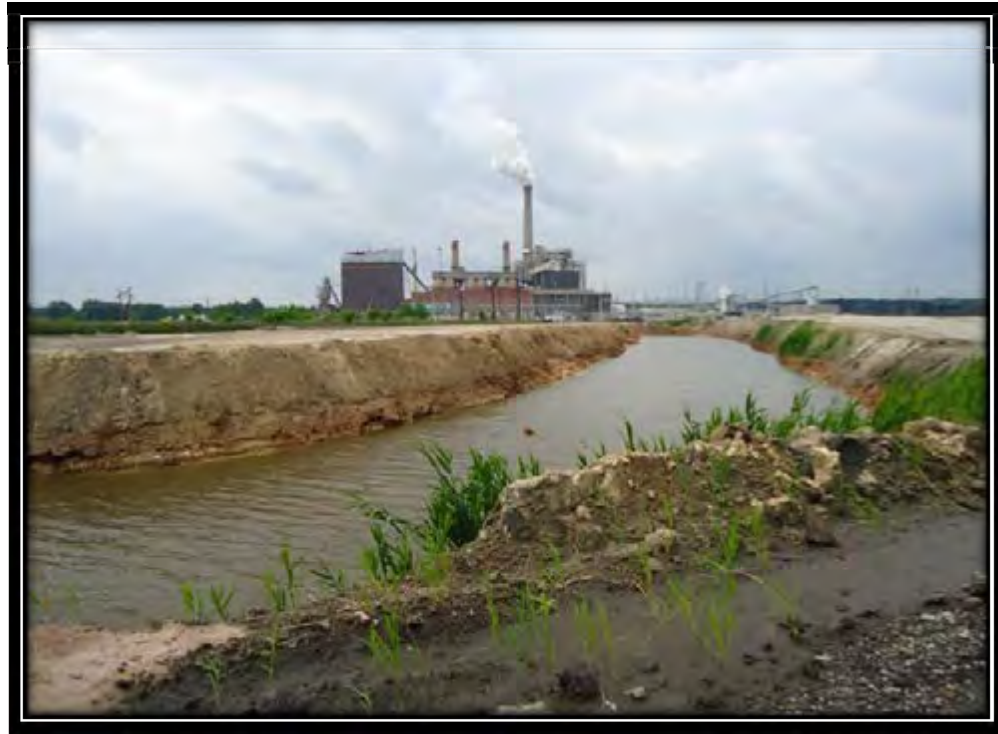
Photo 3 – Pond S-1 General Conditions Photograph
