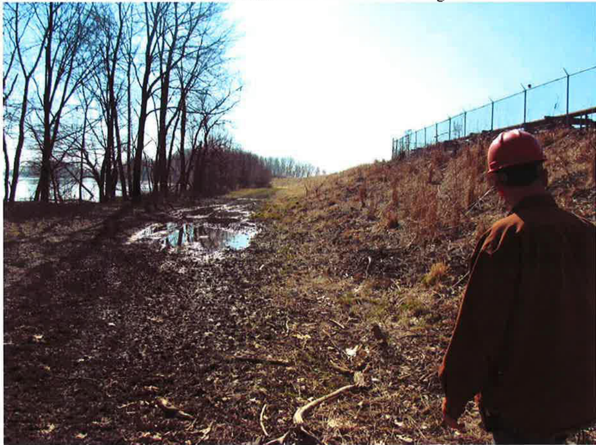
Photo #13 – Bottom Ash Pond - East berm looking south
