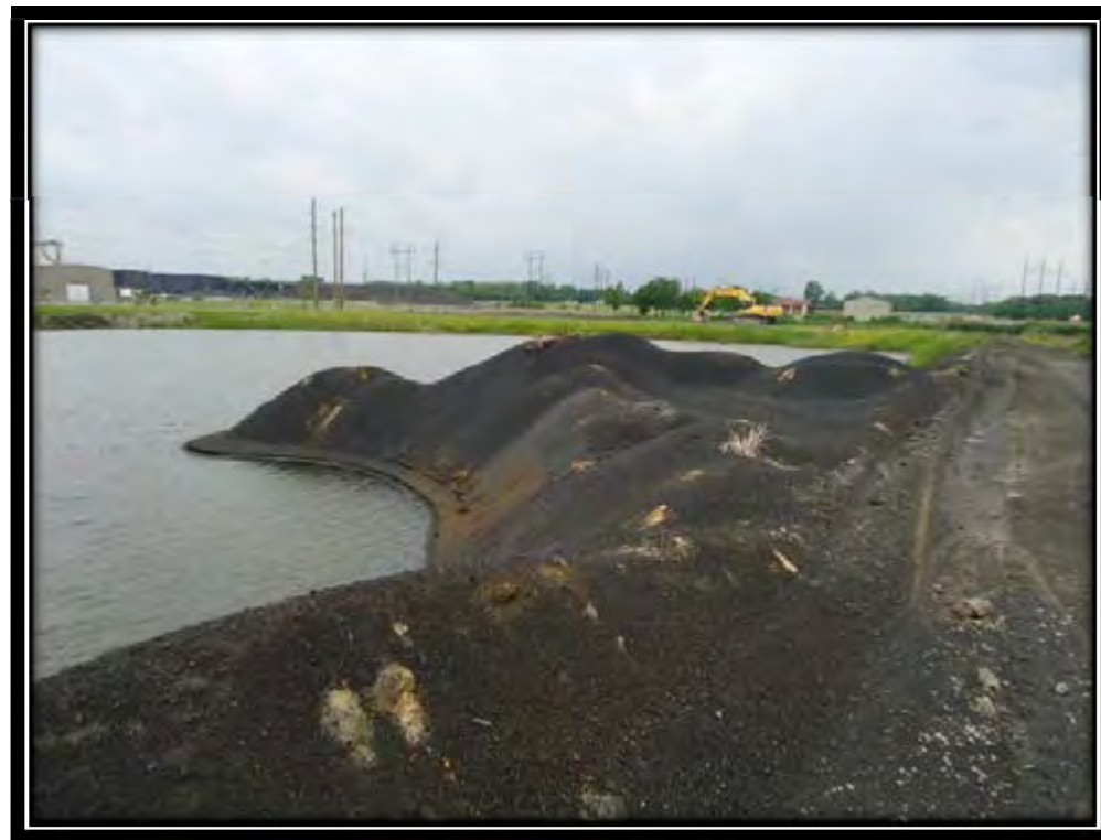
Photo 12 – Ash Pond 1 General Conditions Photograph May 25, 2011 IL50160
