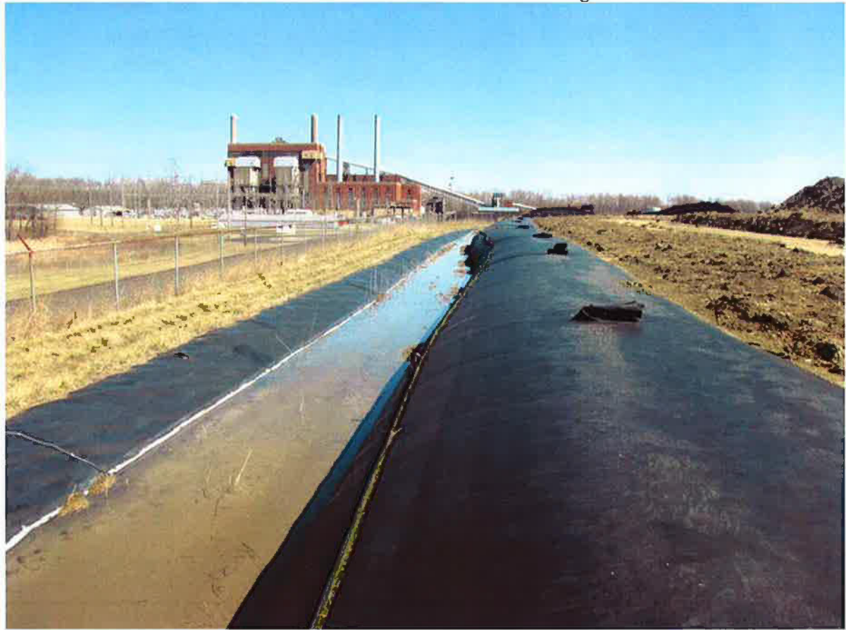
Photo #1 – Ash Pond A – North berm looking northeast
